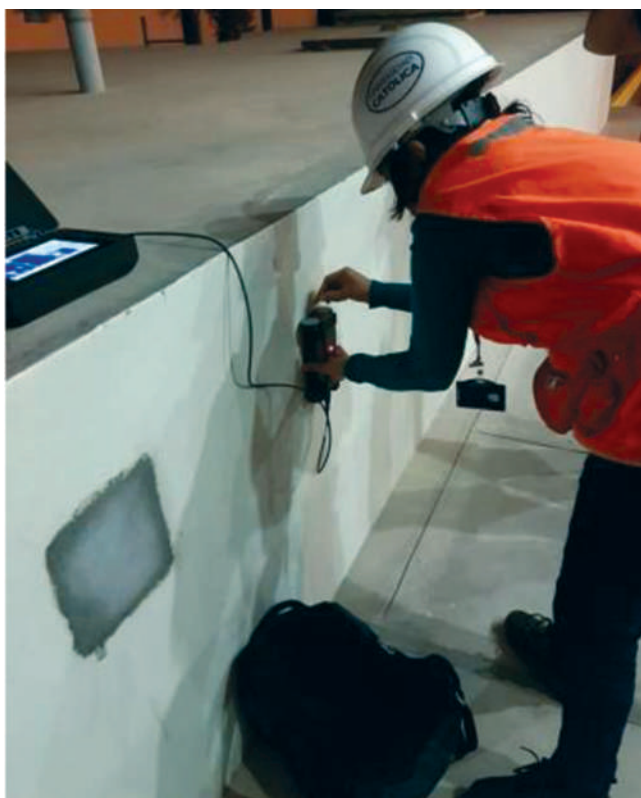
Fig. 21—Wall scan of cistern.
